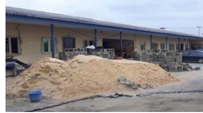
Plate2: Maintenance work at Central Hospital Ugheli
