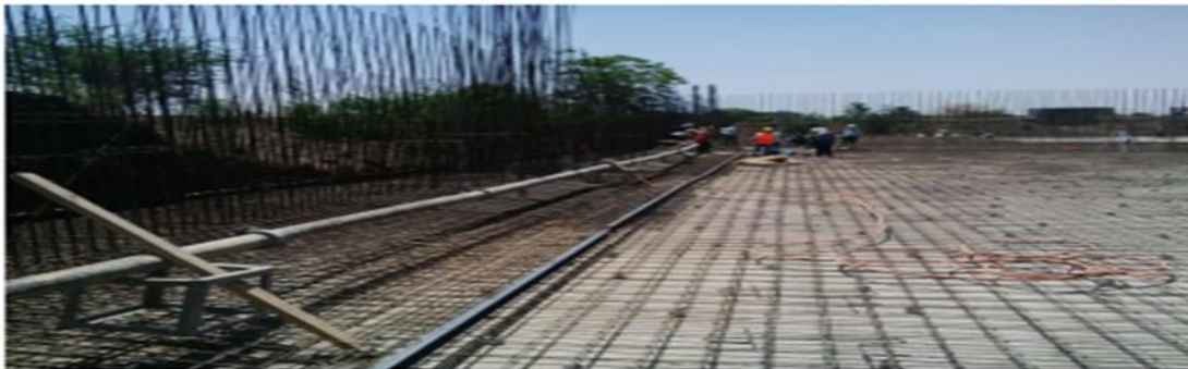
Fig 6.2 STP Slab Casting
