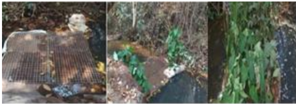
Fig No 8. Construction of Reed Bed
