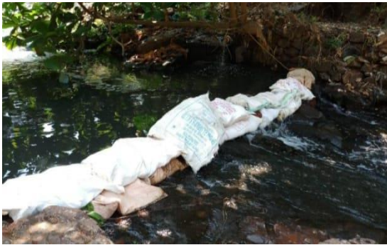
Fig No 2. Construction of bund1
