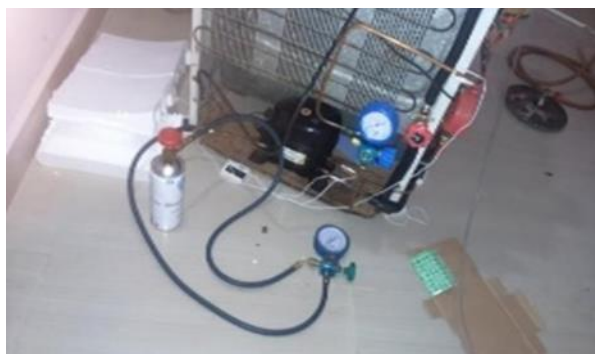
Figure: Gas Charging
