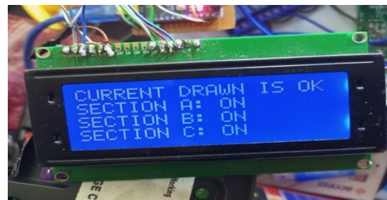
Figure 8a: All loads ON when the current drawn by each section is within the range.
