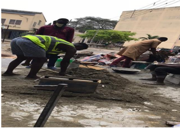
Fig 1: Mixing of hollow block materials for casting
