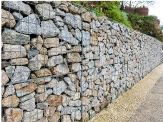
Image:- Weldmesh Gabion Wall
