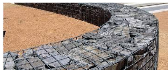
Image: -Curved gabion walls
