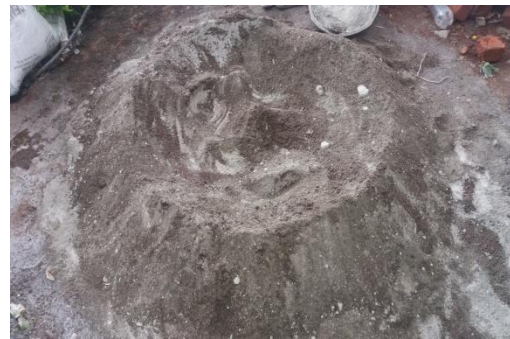
Fig.1 Dry Mixing of mortar with GBS
