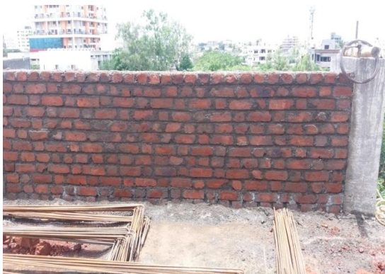
Fig.4. 40% GBS substituted mortar used for Brick work
