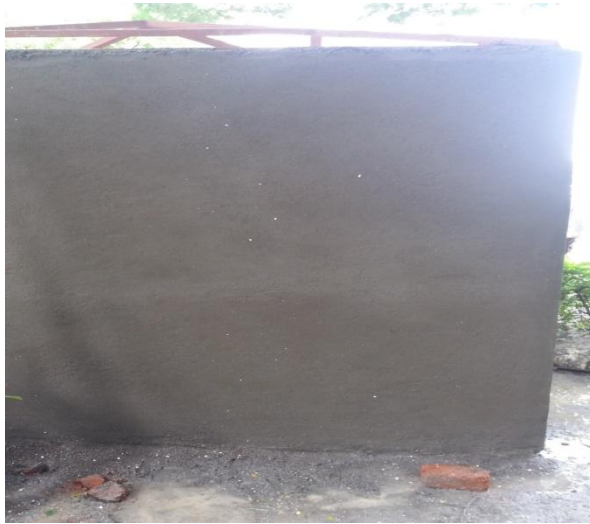
Fig. 3 Finish Surface of plaster
