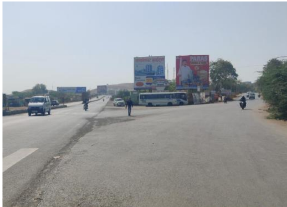
Image: - At Km. 59+600 (Near Shirur Bypass End)
