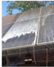
PRESSURE JET CLEANING REGULAR CLEAN PANEL PRESSURE JET CLEANING PRESSURE JET FOMING PANEL SCRUBBING
