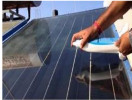
Hydrophobic Nano-coating application on Solar Panels as pre-treatment before regular washing and cleaning
