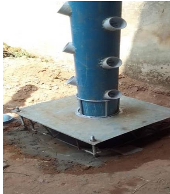
Figure 6: Fixing of the aeroponic stand to withstand wind loading
