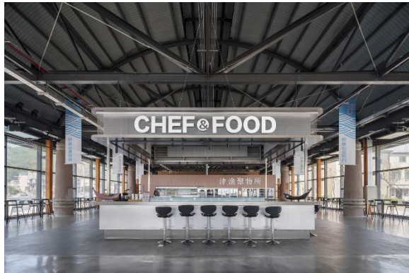
Interior view showing the roof members, double glazing and monolithic finish flooring
