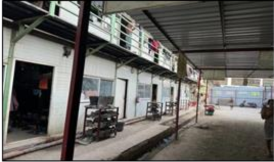
Workers Camp – As per standard practice
