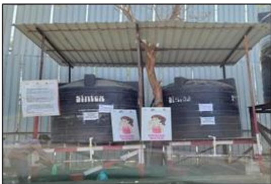
Drinking Water Facilities – As per standard practice
