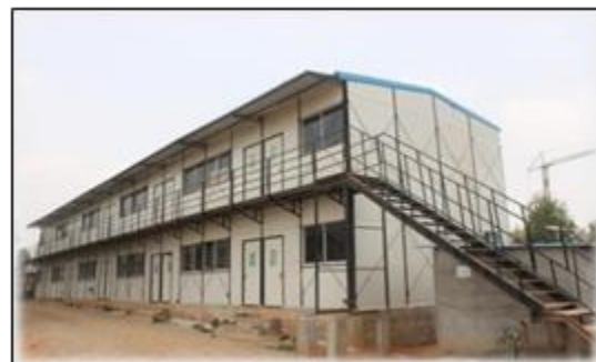
Workers Camp – As per standard practice
