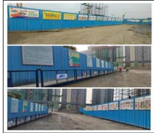
Project Site Barricading
