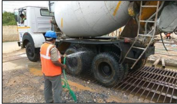
Dust Control at Site – Wash Bay as per standard practice
