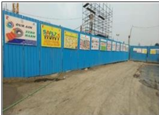
Project Site Barricading
