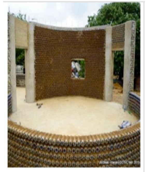
Figure 2: Plastic bottle construction in Yelwa, Nigeria. Source: Hattam (2011)
