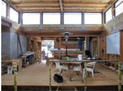
Fig 3: Showing Clerestory Windows. (Source, Pinterest, 2016)
