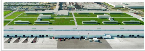
Figure 2: Ford Plant Green Roof
