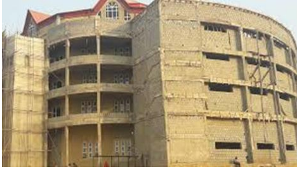
Figure 5: Exterior view of the city of wonders under construction
