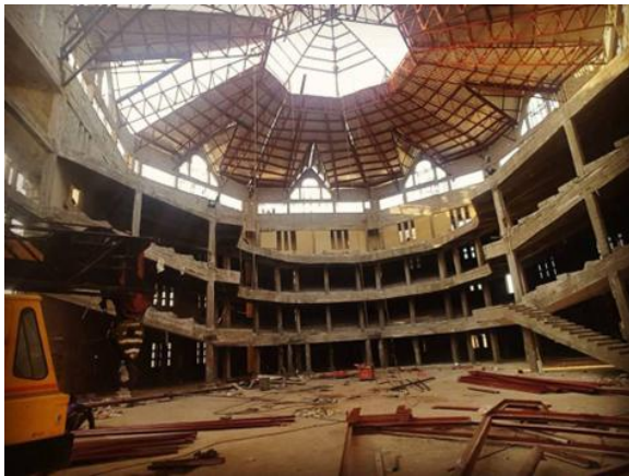
Figure 5: Interior view of the city of wonders under construction
