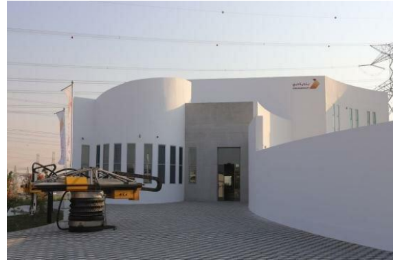
Figure 4: The 1 st (around the world) two story 3D-printed house -Dubai (Al-Qudaih & Sevim, 2016).
