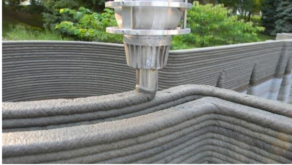
Figure 2: Jetting of the printer ink (Al-Qudaih & Sevim, 2016).
