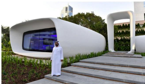
Figure 4: Office building in Dubai printed by WinSun (Ghaffar, Corker & Fan, 2018).
