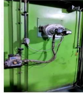
Fig 2.6: Lehr oven burner attached to the body of the lehr.
