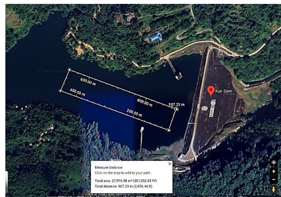
Fig. 2. Installed PV System Area on Kun Chaung Dam
