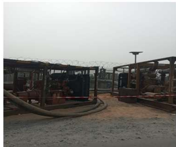
Plate 1b: Oil Well Activities and Facilities in Oloibiri Community, Ogbia LGA, Bayelsa State
