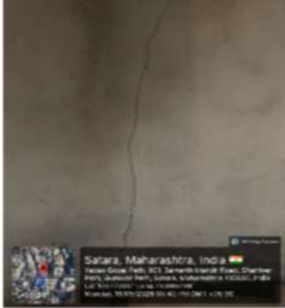
Fig.5. Original Crack
