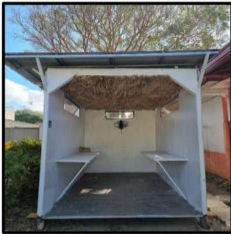
Fig. 3. Actual prototype of the developed mobile study shelter with banana fiber roof insulation.
