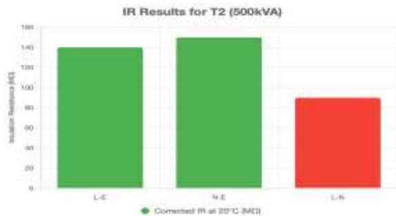
Fig. 10. IR test results for T2 (500 kVA) the L-N configuration (red bar, 90 MΩ) falls below the IEEE 100 MΩ minimum threshold, indicating localized insulation degradation (FAIL).
