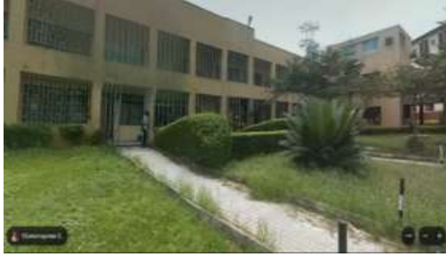
Figure 8: A Site Layout and Photography from the Courtyard.
