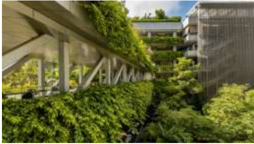
Figure 8: Photos showing verdant greenery from the rooftop to the basement, giving Khoo Teck Puat Hospital its hospital-in-a-garden therapeutic experience.
