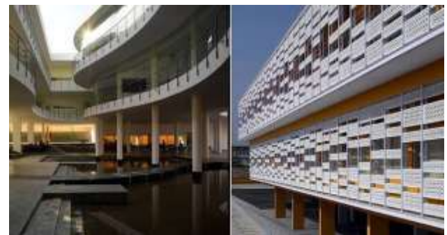
Figure 10: Photos showing open courtyard, stepped well or baoli, and perforated stone screens or jaalis.
