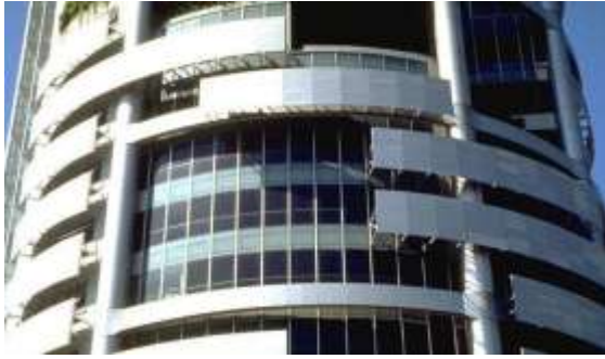
Figure 6: Façade detail showing terraced garden and aluminium screens
