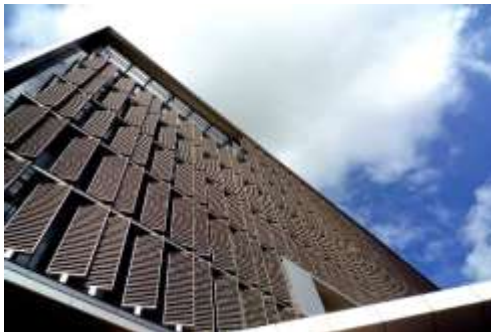
Figure 9: Photos showing the central garden courtyard with water features and façade detail showing louvers.
