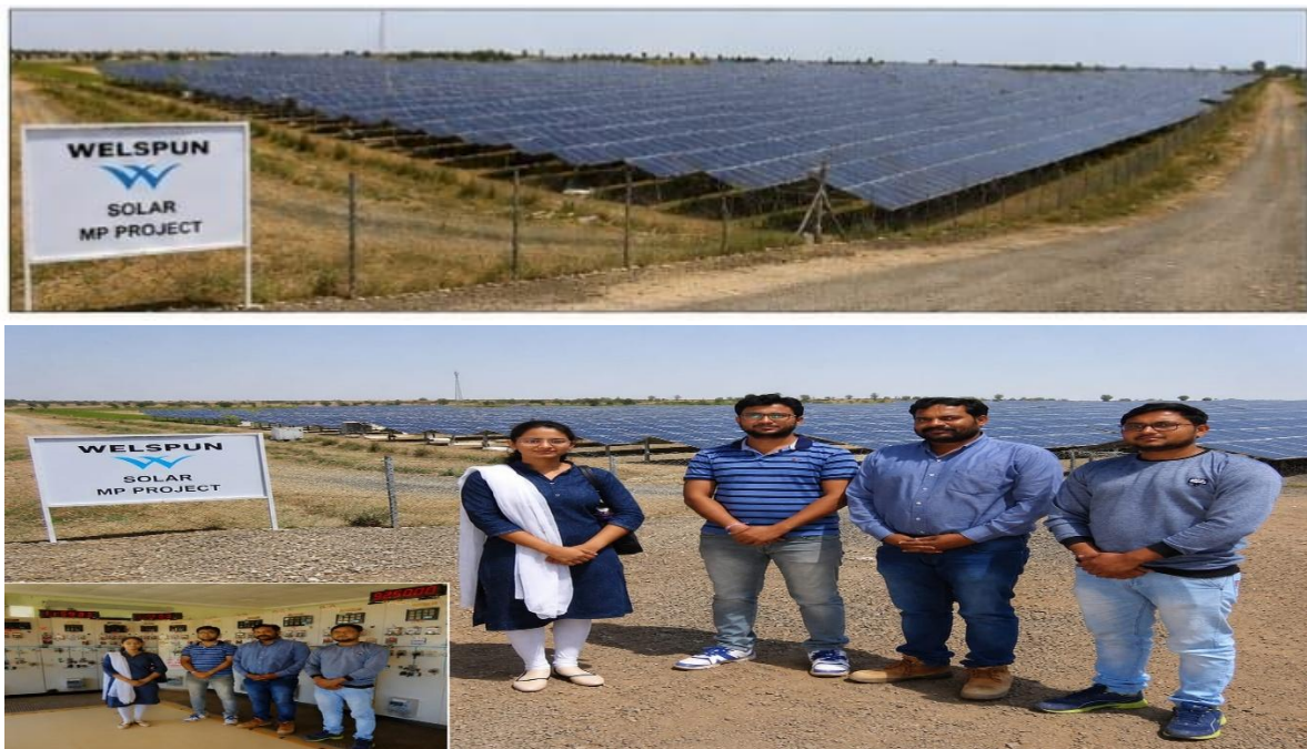
Figure 10.1: Site visit at Welspun Solar MP Project, Bhagwanpura (Near Diken), Neemuch, Madhya Pradesh. Source: Author's field visit.
