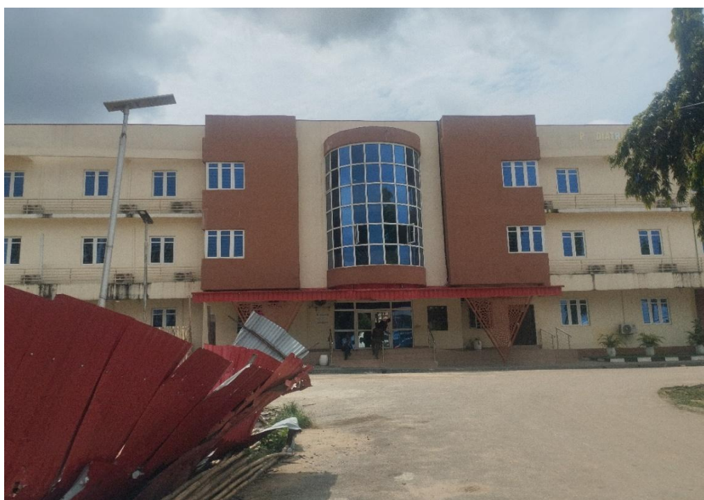
Plate 3: Approach View showing Building Materials of Paediatric Sick Cell Centre LASUTH Ikeja. Source Paediatric Sick Cell Centre LASUTH Ikeja. (2025)
