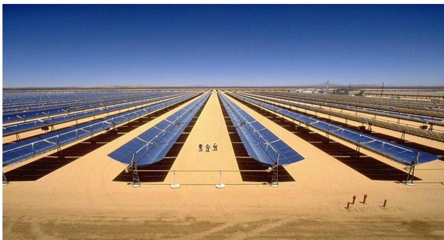
Figure 4 Mojave Solar Project in California showing the parabolic trough solar collector field.
